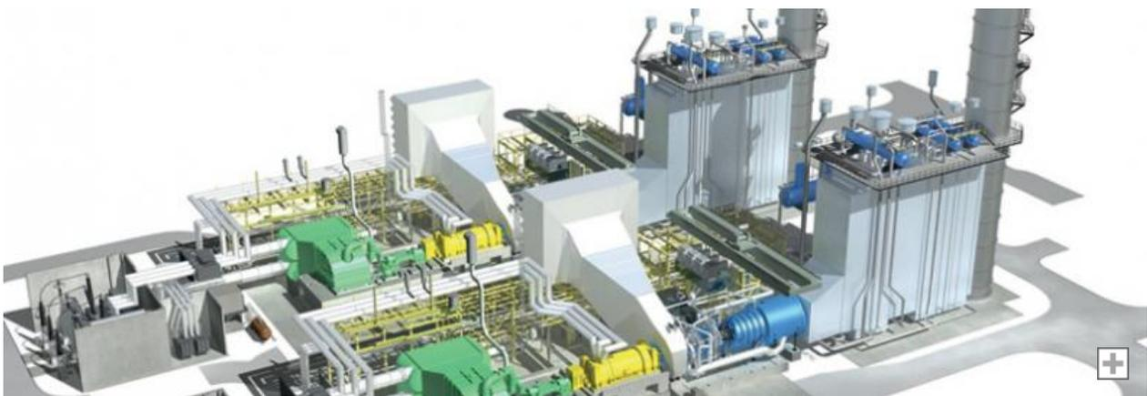
This station is among the best performing power plants in the world with low  $\text{NO}_x$ ,  $\text{SO}_2$  and  $\text{CO}_2$  emissions. It features a high operational flexibility, since it can run at base load and part loads as well as in two-shift operation mode. It is designed around two GT26 combined cycle modules rated at 435 MW each for a gross output of 870 MW at 59 % efficiency.
