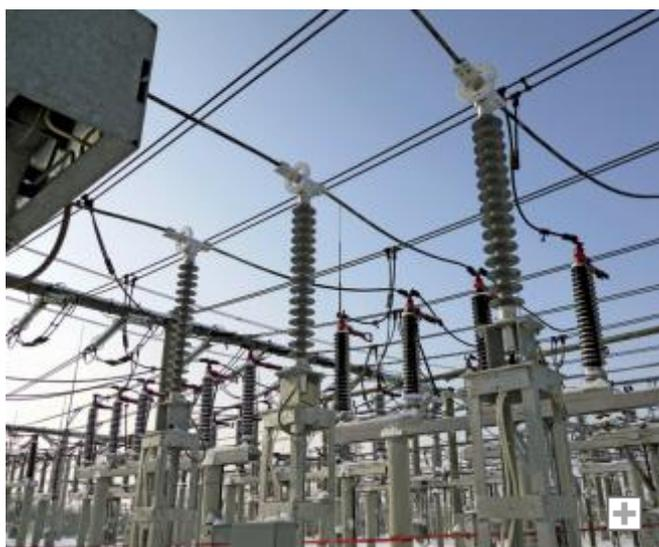
In addition, NCITs feature a high measurement bandwidth for fundamental frequency, harmonics, inter-harmonics, sub-harmonics, and quali-metering (metering of power quality). Another significant benefit is that the NCITs are compact and light in weight. According to Chatrefou, improved safety is a key advantage of the design. “Insulating secondary equipment from high voltages by using fibre optics means higher safety for substation personnel. Removal of wired cross-site current
